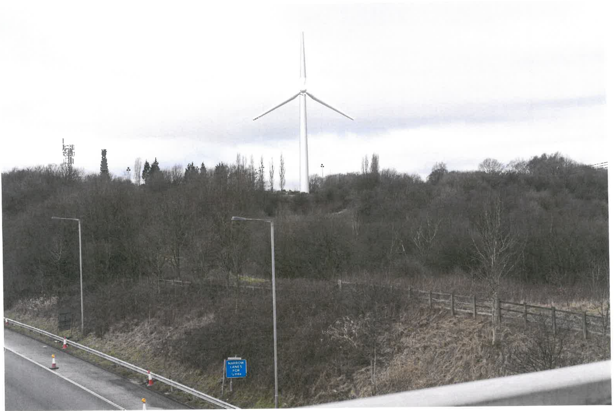
Viewpoint 8: Footbridge Over M60
